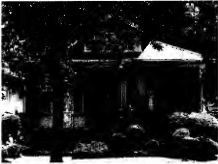
Figure 5: 7527 South Merrill Avenue
